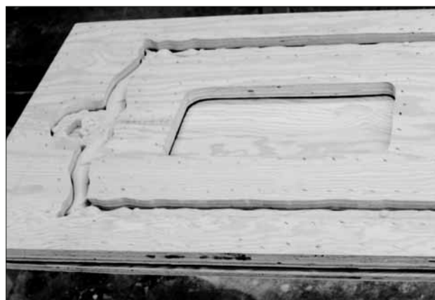
Photo 2: The frame pattern is placed within plywood forms.
