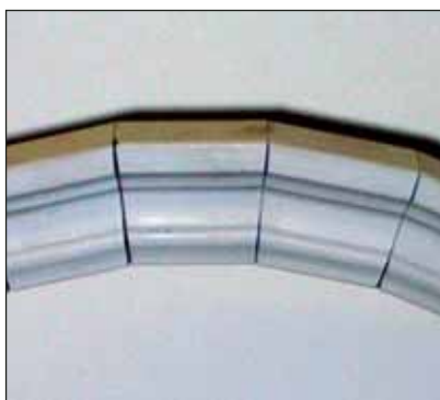
Photo 3: By calculating the correct angle to cut each piece of the angled frame, they were able to be pieced together.
