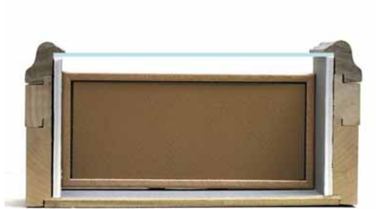
Diagram F: Cut a matboard to serve as the final covering for the shelf. The matboard will cover the nails and give the shelf a clean finish.
