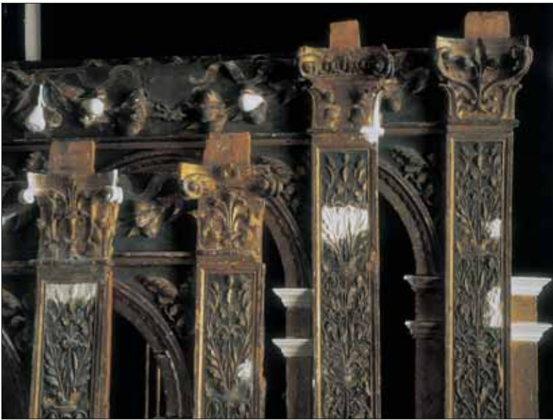
Many small pieces of ornament had to be repaired, replaced, or restored. The repaired areas here have yet to be finished. (Photo courtesy Gold Leaf Studios.)
