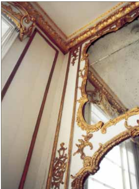
Clockwise from above: This corner of the room shows the many mouldings, mirror frames, and the wainscoting that needed repair. Annie and Francesco Gronchi, who were trained on this extensive project. Some areas has more missing than existing ornamentation.
