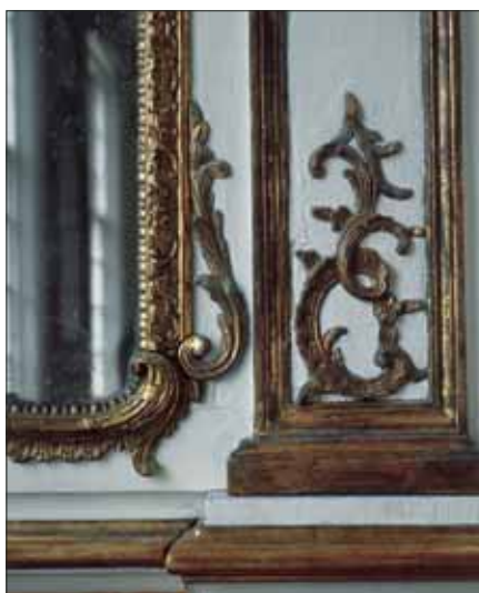
Two dominant styles of Louis XIII and the Regence period co-exist in silent symbiosis within the room as a unified whole. Shown after intense conservation efforts, one contains an intensely deliberate cross-hatched gesso as a background pattern for small "C" scrolls that terminate in a roccaille shell/leaf pattern. The other has a relatively simple ogee molding that still has the flourishing terminal Rococo leafage as counterpoint to the plain moulding.
