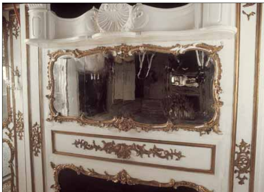
One of the many mirror frames, with white (ungilded) areas showing necessary repairs.
