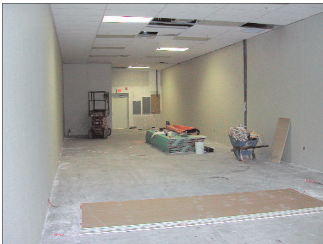
... A month before moving in—buildout proceeding...
