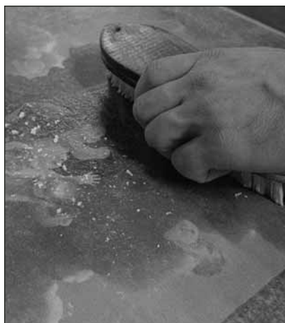
Photo 4: Any remaining paper can be removed by scrubbing with a brush.
