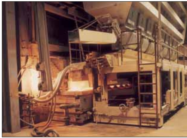
At the “hot end” of the float line, the ingredients for glass are loaded and melted. This begins the manufacturing process, which results in sheets of glass at the end of the line.
