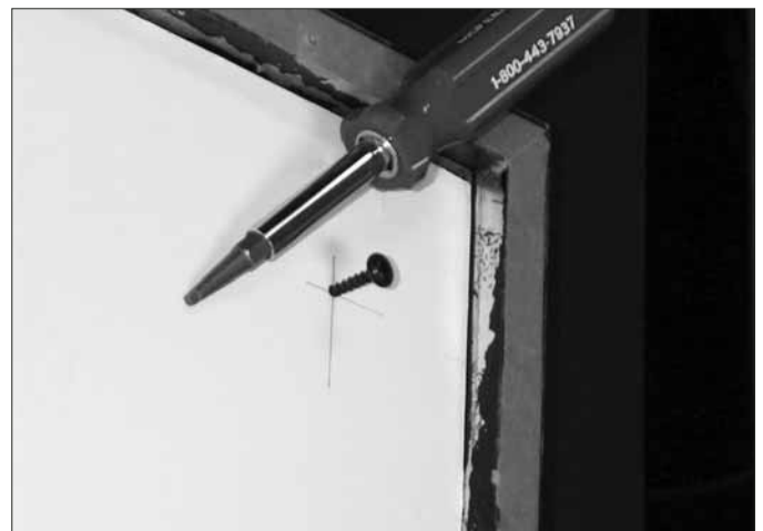
Photo 2. The screw hole can be enlarged to ensure proper placement without being visible due to the large incorporated washer head.
