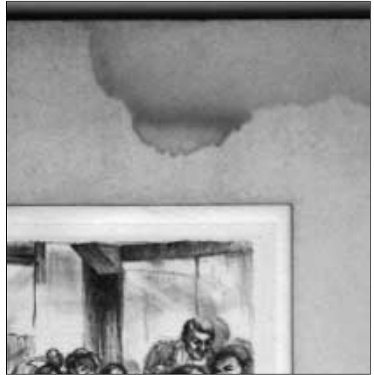
The water damage on the matting of this frame package threatens the artwork. It was not framed preservationally, and should be reframed to ensure its longevity.
