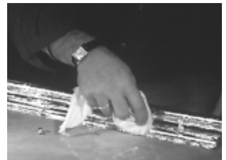
A rag is then used to wipe down the frame.
